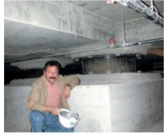
Farzad at the base of Los Angeles City Hall after it was retrofitted with a complex base isolation system to enhance its earthquake safety. One of the isolators is apparent behind him. Farzad was the chair of the peer review committee for the project.
