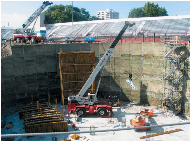
USC's new thermal energy storage system under construction in Cromwell Field.
